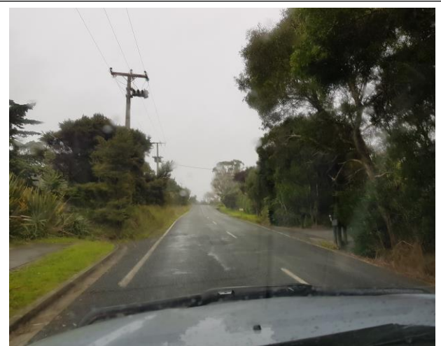
Figure 4: North end of Old Waipu Road
