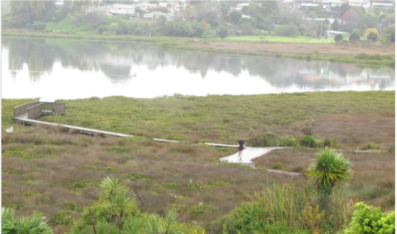
Figure 17: Tauranga City Estuary Board walk 1m above estuary level 2m wide.
